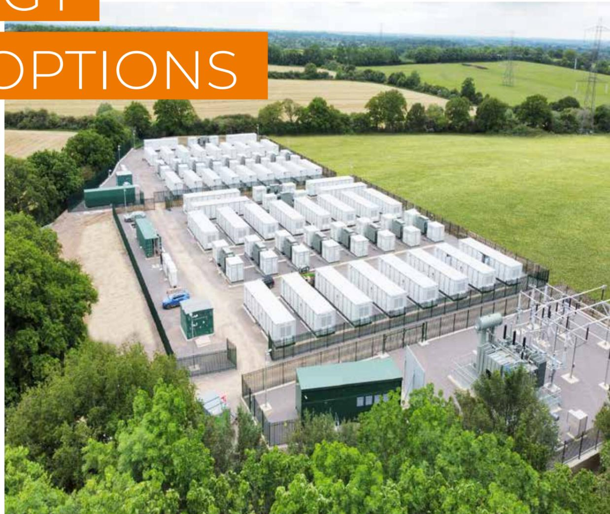
**The largest unsubsidized grid-connected standalone battery storage plant in Europe: 100MW/100MWh**
